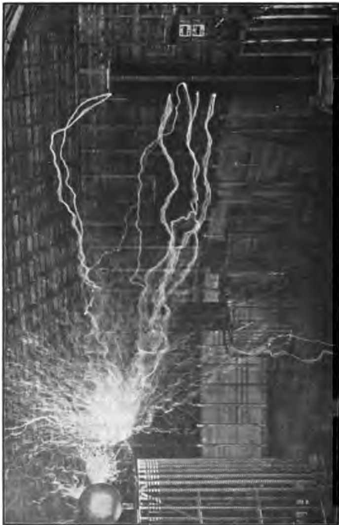
FIG. 176.—EXPERIMENT TO ILLUSTRATE THE CAPACITY OF THE OSCILLATOR FOR PRODUCING ELECTRICAL EXPLOSIONS OF GREAT POWER.
