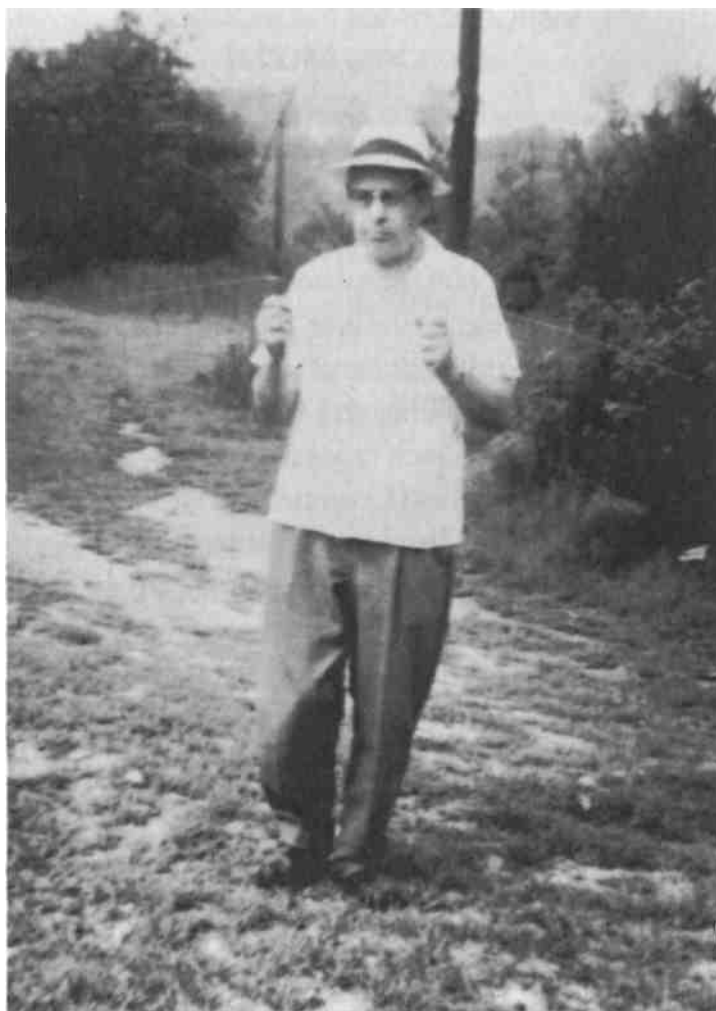
Figure 2-1: Employee of the Milford, Connecticut, water company using detector rods to locate city's water mains. Employee did not wish to be identified nor would he permit a second photo session.
